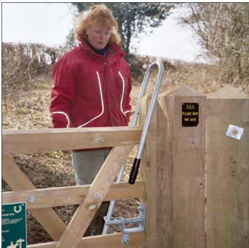
*LHA PROW officer checks the installation of a new wooden one way self closing 5ft gate at the Murder Combe bridleway entrance off the highway before the route is opened to the public. Note that the gate slams against the boundary and a Centrewire easy trombone latch has been installed along with a 'please shut the gate marker' and a sign detailing who dedicated the route and who funded it.*
