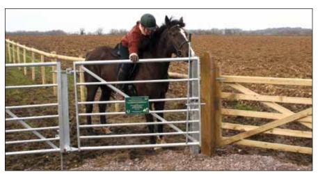
Dual-purpose Centrewire York gate at Murder Combe with a two-way opening bridleway gate and integral vehicular gate section that can be locked to prevent unauthorised use. A new entrance into this field has been created (on right). The stock-proof fencing erected has barbed wire on the field side but the horse and rider are protected by the rail on the inside.
