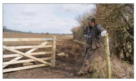
TTT's contractor installs furniture on the Murder Combe route. This additional gate was installed to provide the tenant farmer with a new entrance to his field as the original entrance was fenced off to facilitate running a new length of bridleway along the field headland.
