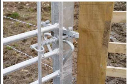
Exit: York bridleway gate with two way catch from Centrewire leads out of fenced in corridor into green lane. Integral field gate section can be locked to prevent trespass by vehicles.
