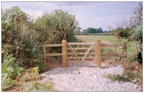
Section of community trail at Binegar (see TTT case study 2, guide section 23). This new bridleway at Rookery Farm crosses land where horses and cattle are kept and is close to a busy main road. It has been fenced with posts and inner top rail and field side stock proof fencing to form a safe user corridor to seperate users from stock and to ensure stock security.
