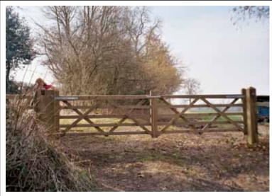
New bridleway entrance from the two track rural road has been constructed. There is ample room for users to enter or exit before or after crossing the road to or from the verge on the other side leading to the Fordbury Lane section of the trail. The barbed wire Wiltshire gate has been replaced with a pair of wooden estate gates plus a 5ft one-way bridleway gate closing against the boundary has replaced the original kissing gate.
